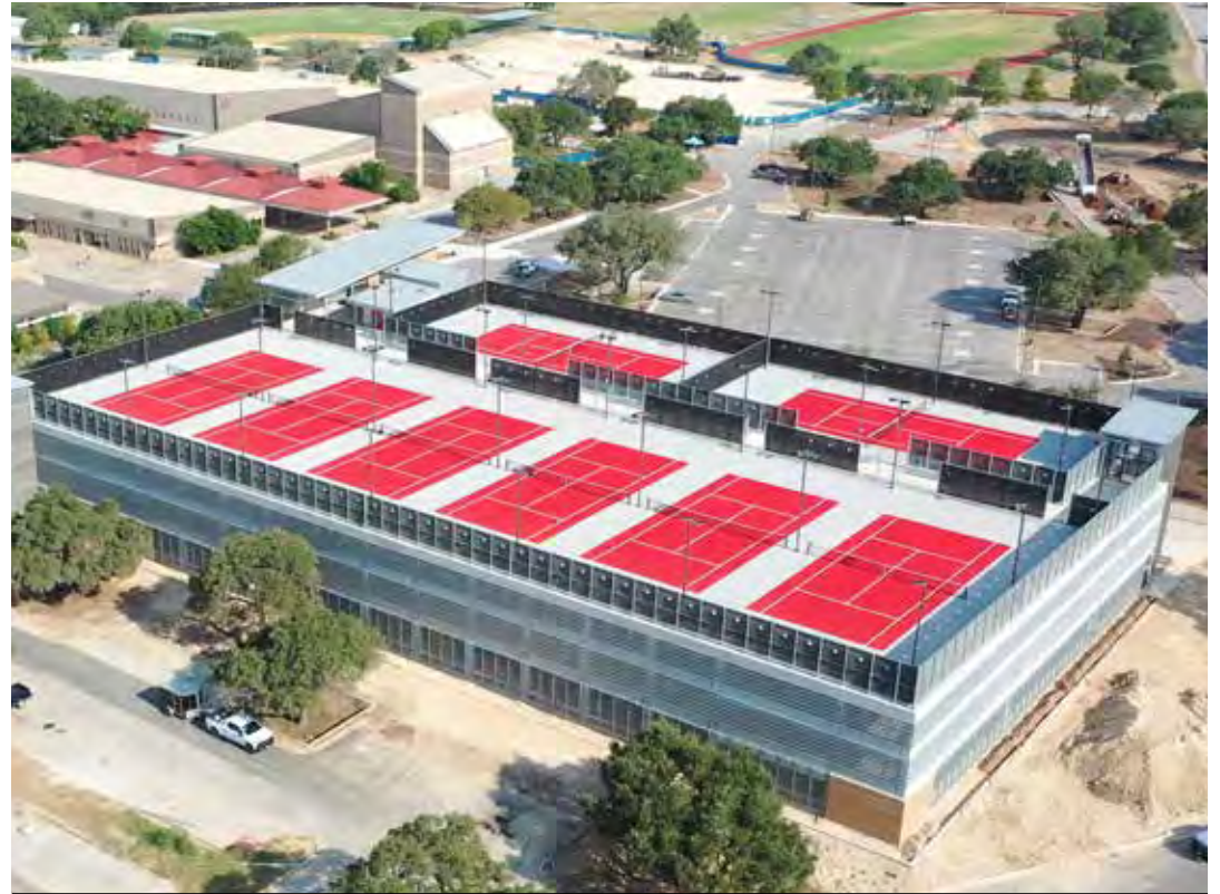
Bowie High School Parking Structure - Featuring Tennis Courts and Marching Band Practice Area, was built to comply with city code requirements for parking and to reduce impervious cover for water quality while modernizing the campus.
