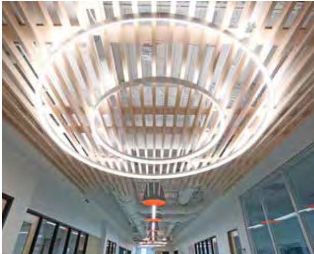
LED Lighting - Saving Energy
