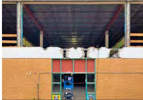
Sánchez Elementary Future Site of Learning Stairs
