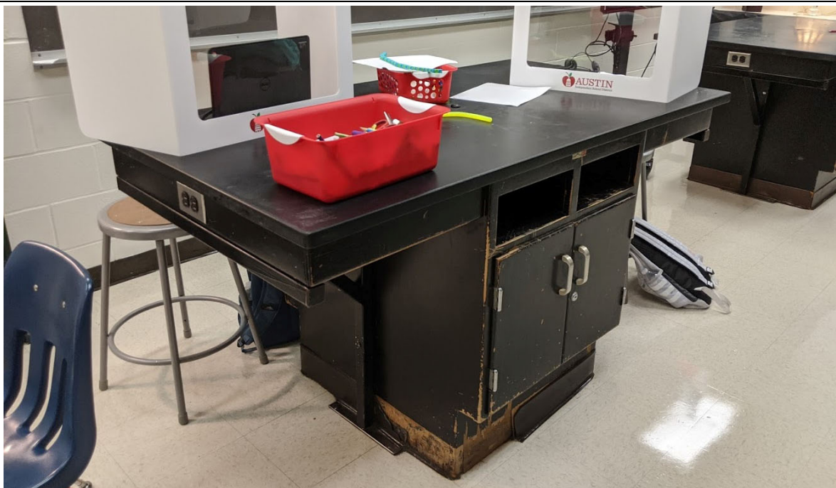
Furniture – Original Lab Tables in disrepair, these are heavy and immobile
