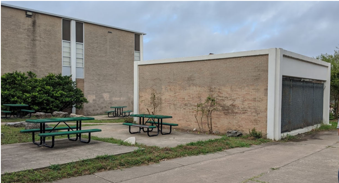
Outdoor Learning – Existing space disrupted by noisy mechanical equipment and no shade is provided.
