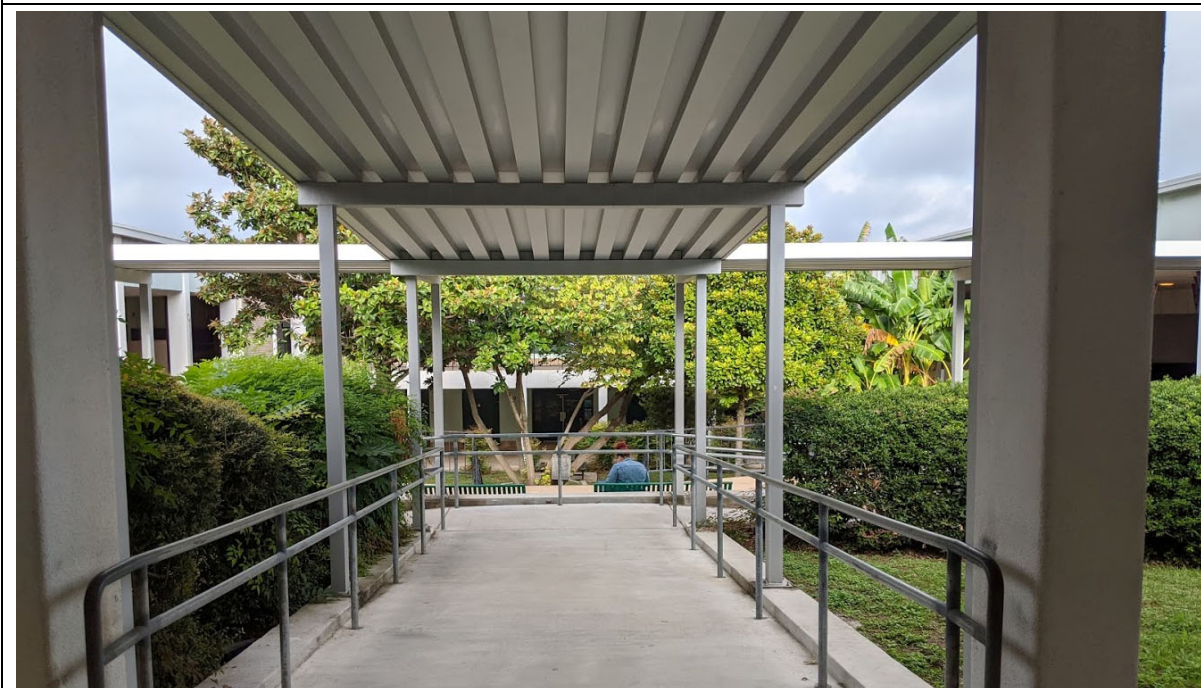
Interior Circulation – Accessible Ramps in Central Courtyard Space
