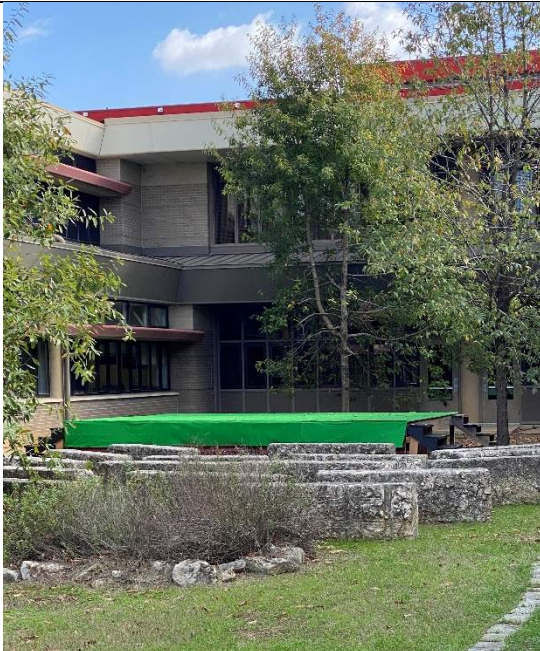
One courtyard in the academic wing contains a solar studio and an outdoor theater. Some trees are mature and provide shade, but more shade (and technological support) is required in all courtyards.
