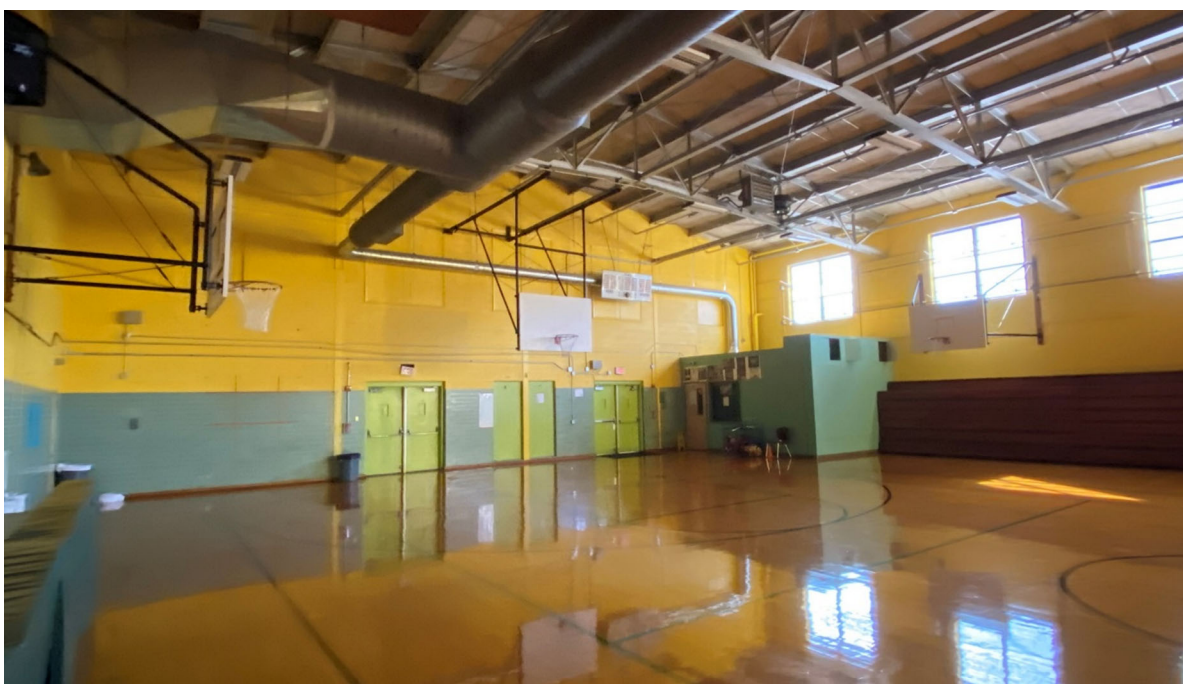
Gym is original to school and has not been updated.
