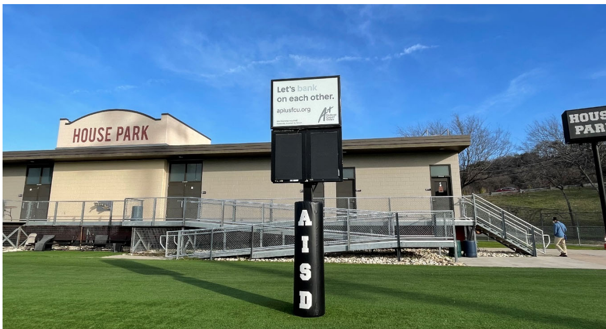
View of Field House. It has ADA access. The building appears in good condition but is deficient in meeting some needs.
