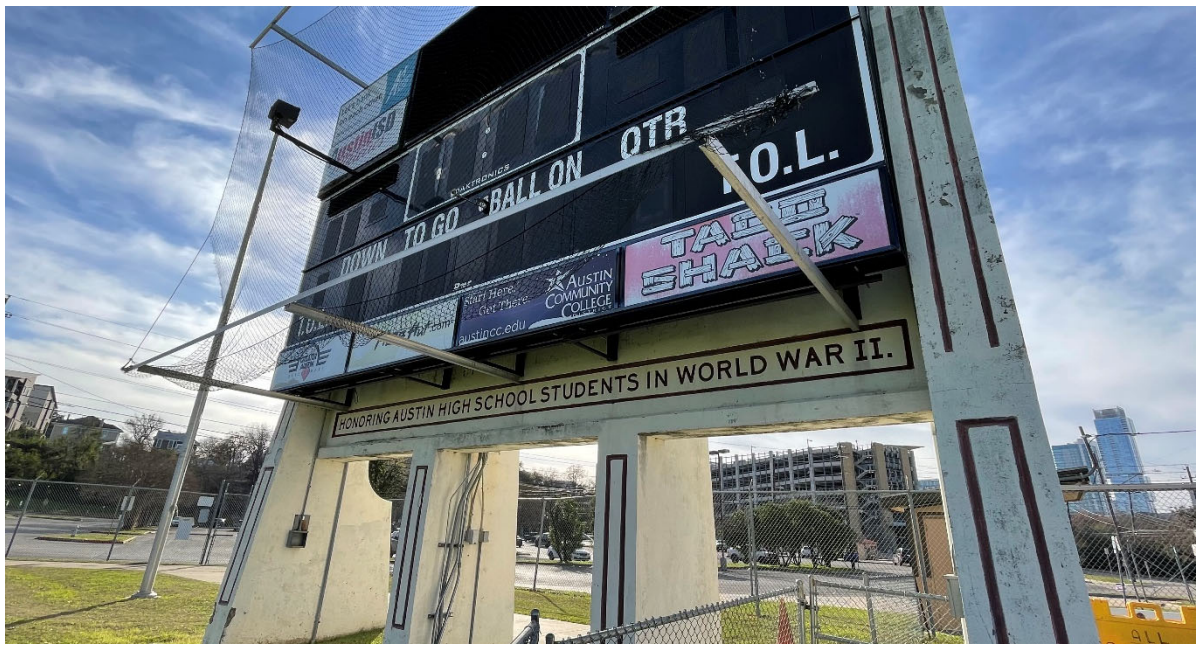
Existing scoreboard has some historic characteristics but needs modernization.
