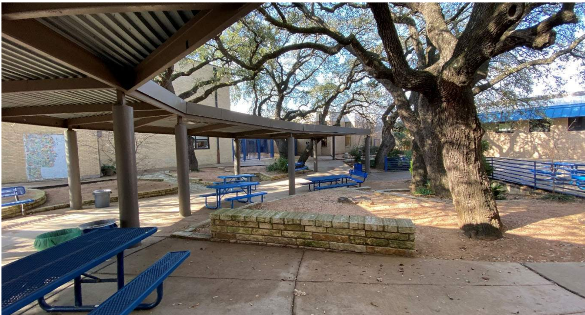
Internal Courtyard: Mature trees provide shade for outdoor seating. There is a covered walkway between buildings. During rain events, drainage issues and standing water (mosquito issues) occur.
