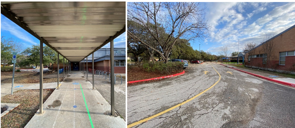
The drop-off canopy needs updates and better lighting (left); the primary entry drive loop needs wayfinding signage (right).
