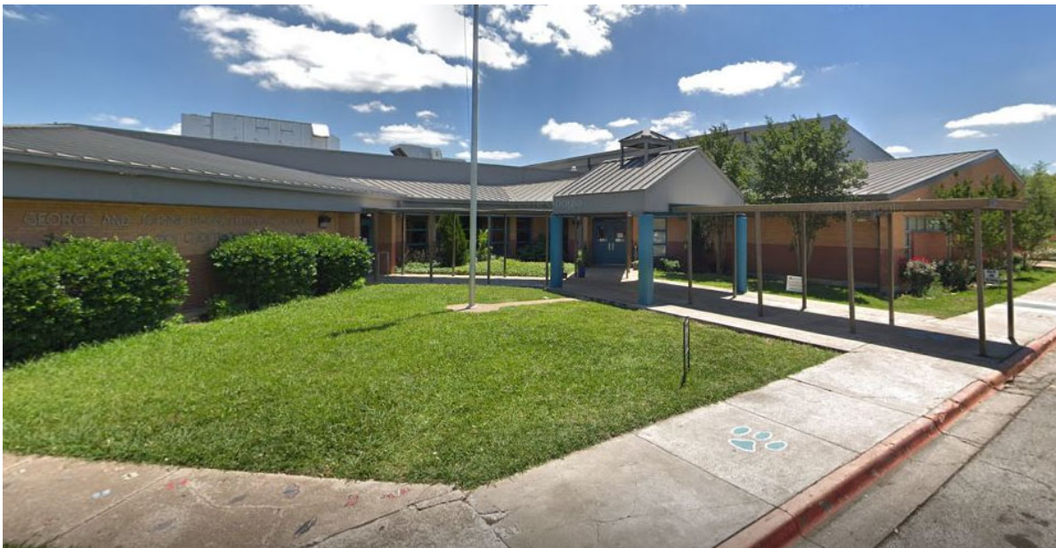
A large, covered walkway provides a welcoming front entrance, but school signage is poor.
