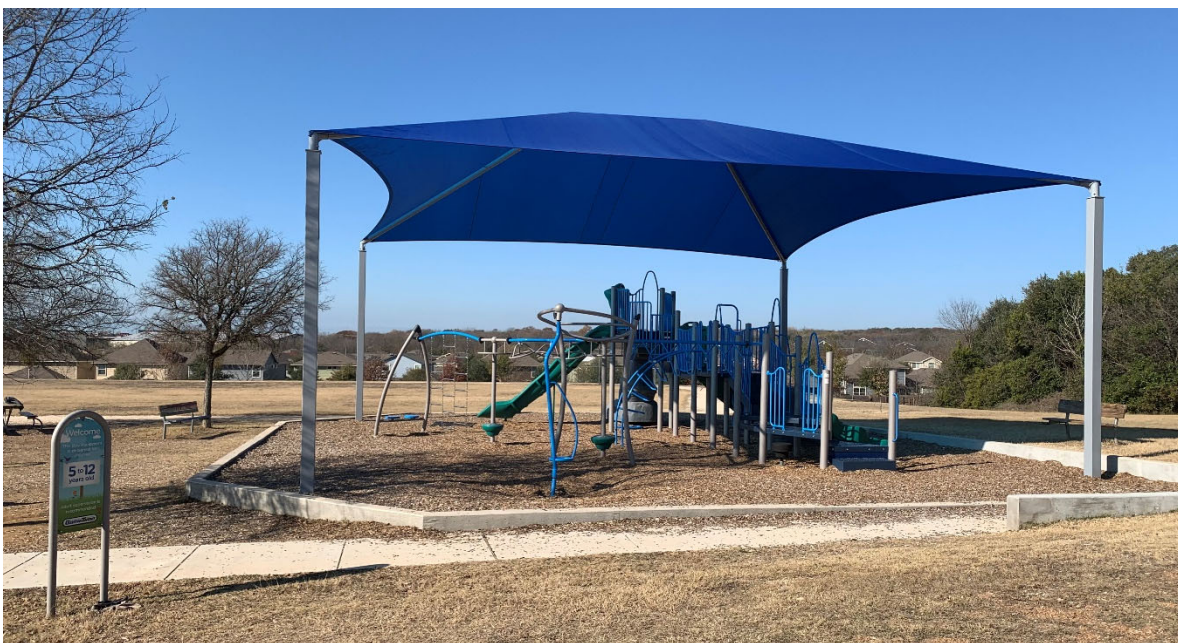
The play area is fully covered and in excellent condition.
