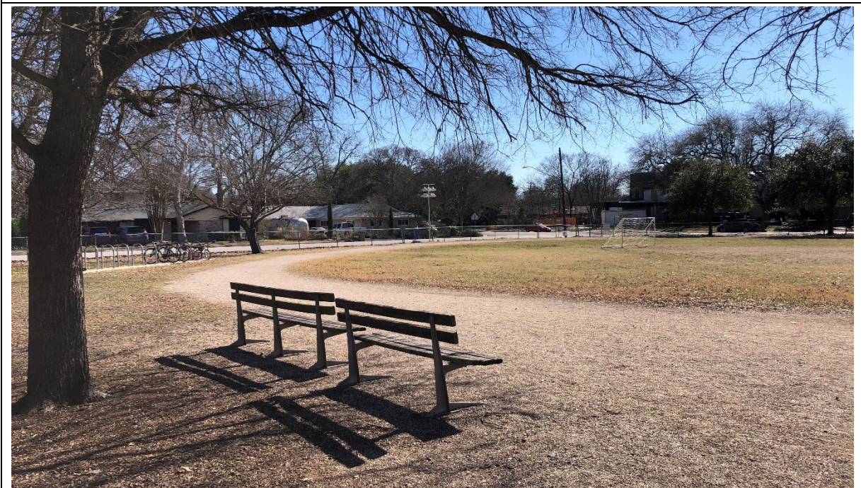
Running track is uneven and creates trip-and-fall hazards.
