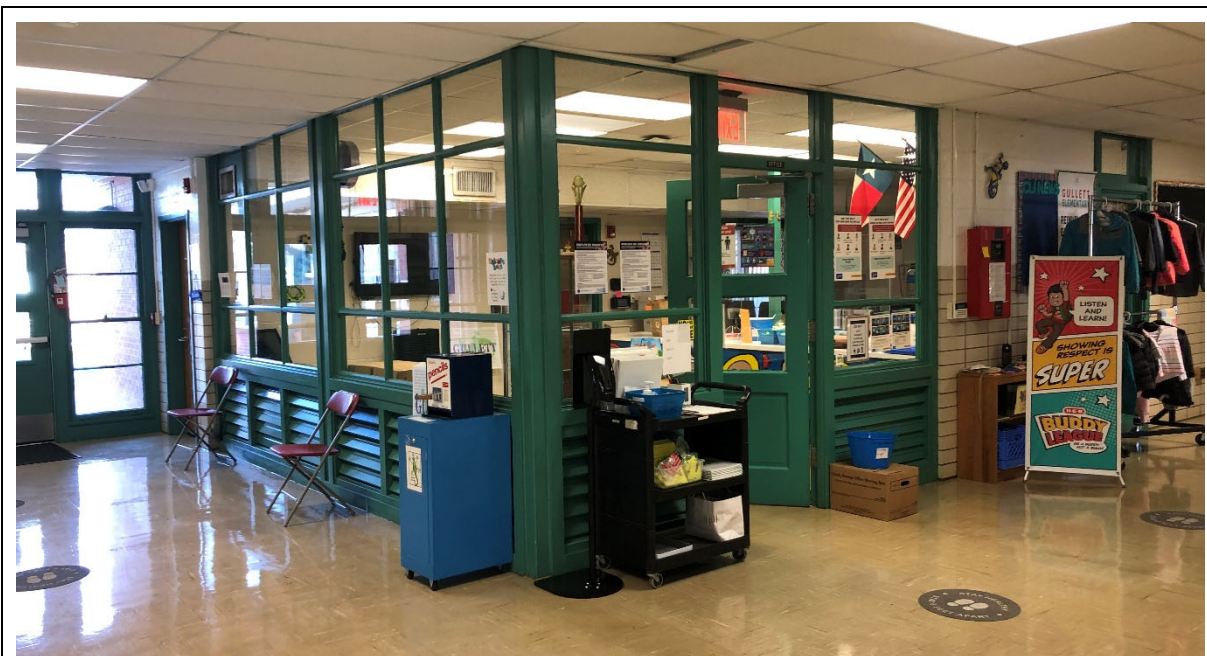
Administration: Main office is located near the primary entry. It is missing many programmatic elements, such as a conference room, staff lounge, separate offices for principal / Asst. Principal, and nurse's office.
