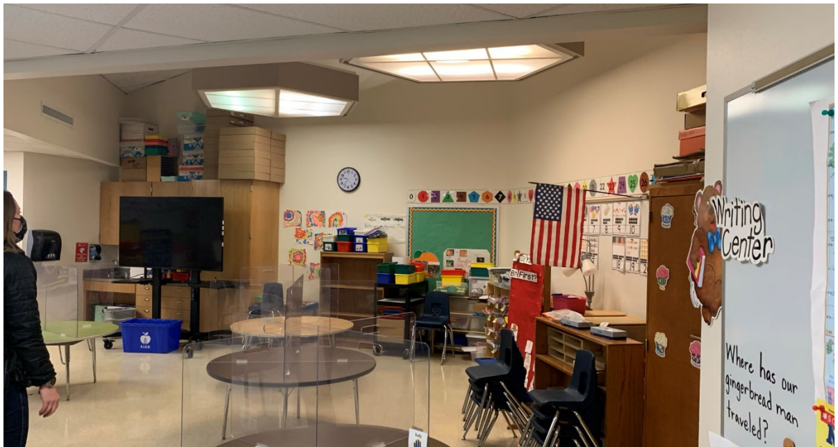
Studio in the interior of the ring. Studio is undersized per Ed Spec and does not have any access to natural daylight and no transparency between the studio and corridor.
