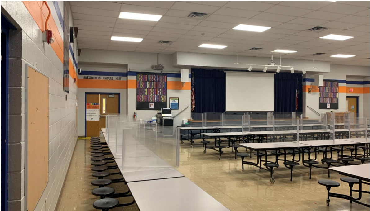
Cafeteria and support spaces are undersized per Ed Spec. Stage is small and ramp is outside of the cafeteria for stage access.
