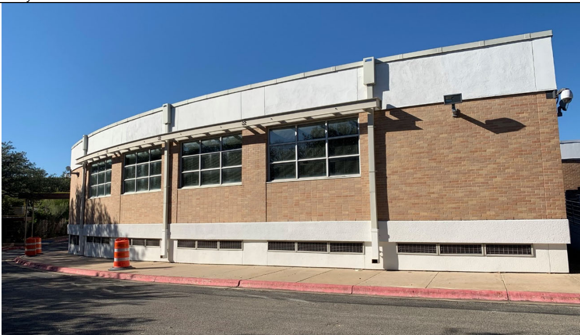
Brick and stucco are in good condition. Stucco was recently painted.
