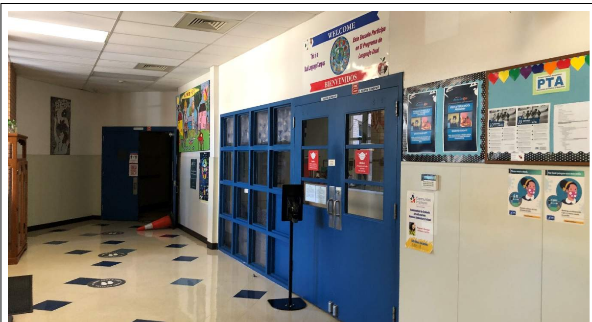
The main entry is not overly generous and not an inviting entry space.
