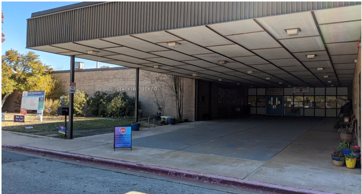
Main entry to the school with large canopy.
