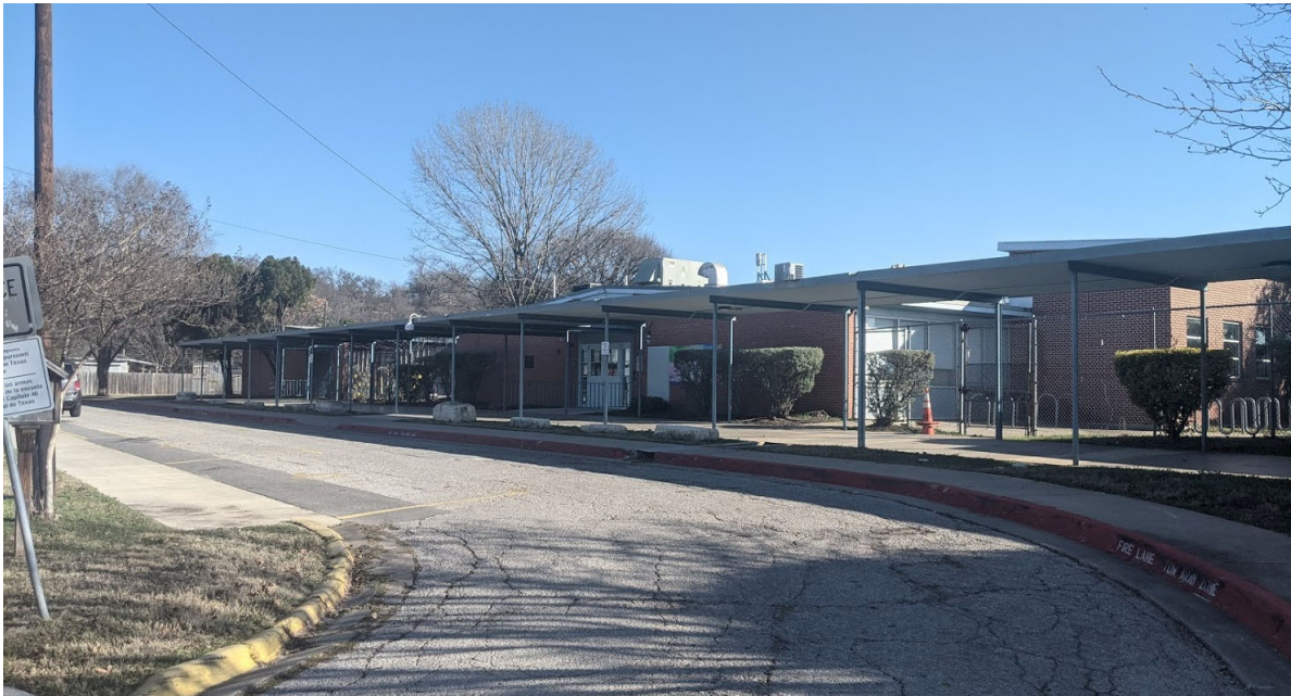
Main building entry provides covered area for pickup and drop-off, but main entry door feels unwelcoming.
