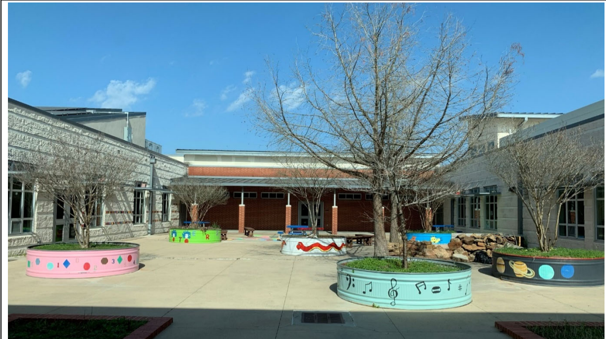
Outdoor Learning and Activity: The internal courtyard with seating, planters and a learning pond (right side of photo).
