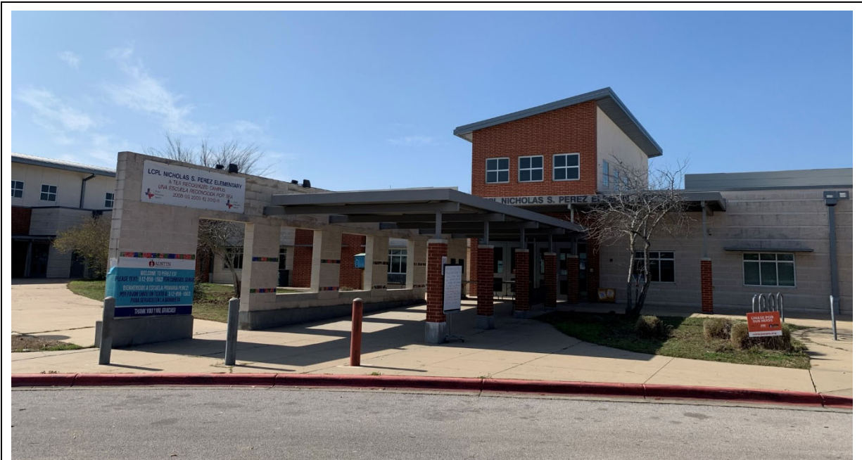
Exterior: Main entrance is easily recognizable. Student work on display under canopy conveys pride for students.
