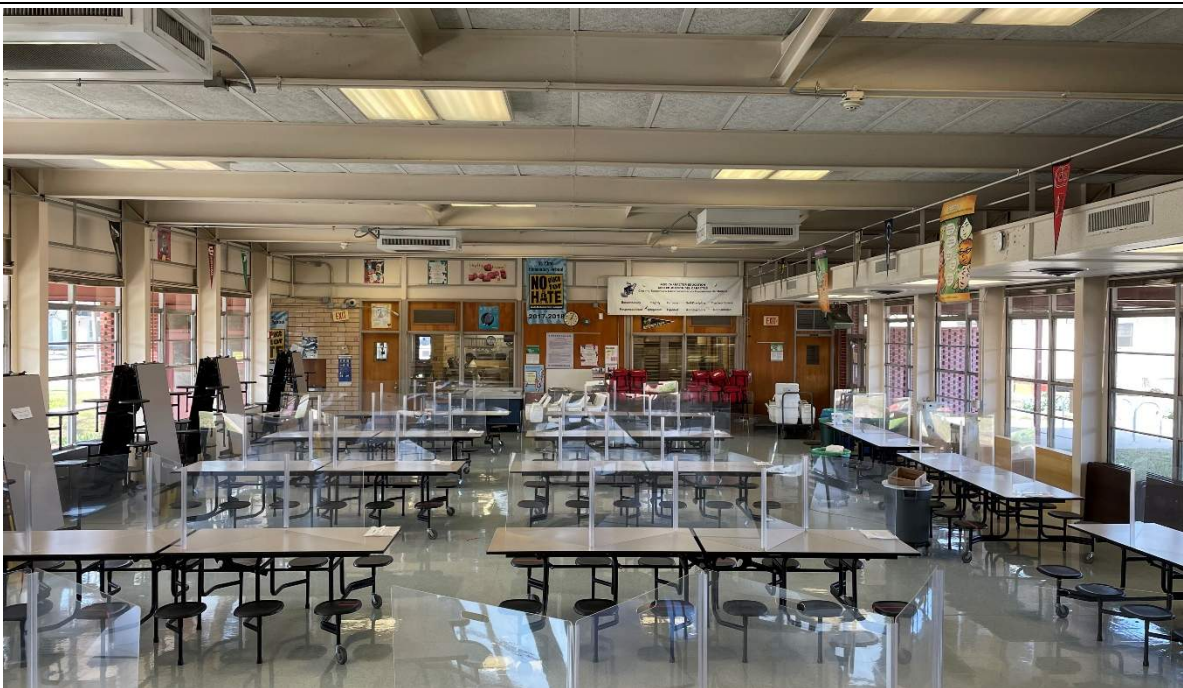
Food Services: Cafeteria is sized appropriately for campus capacity with natural daylight and views to the outdoors provided by windows along both sides.
