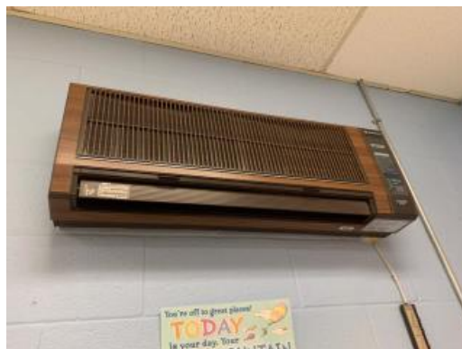
Wall Unit is old and near end of life
