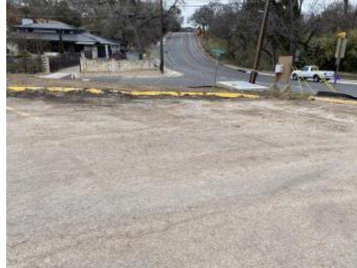
Aged asphalt pavement
