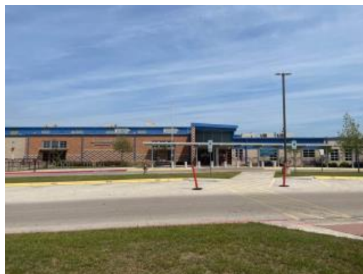
Main Entrance, east elevation
