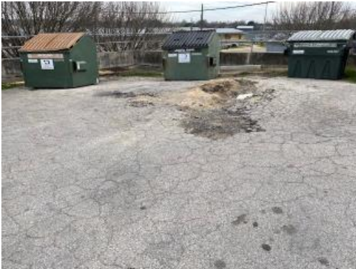
Damaged asphalt
