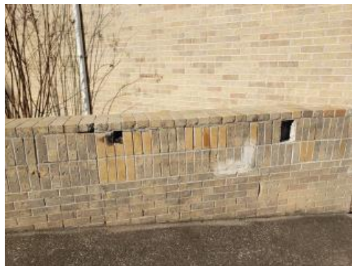
Damaged brick along walkway
