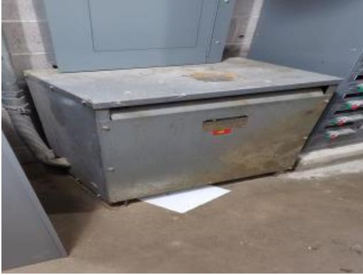
Electric transformer
