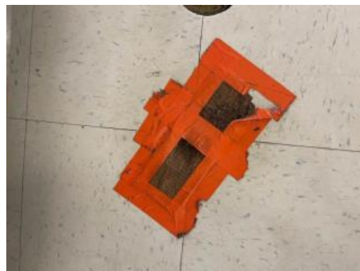
Wear and tear of vinyl composite tile
