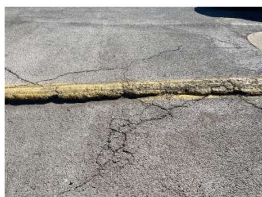
Damaged asphalt
