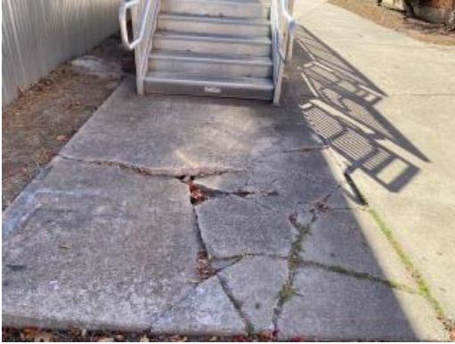
Damaged sidewalk
