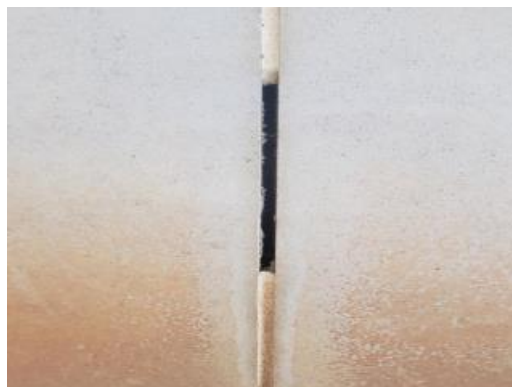
Failing sealant
