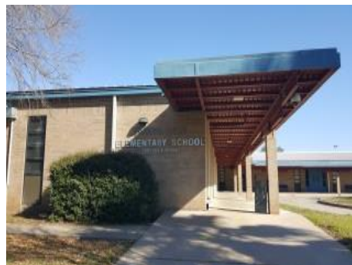
Covered Walkway to School Entrance
