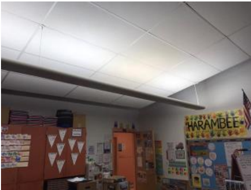
Typical classroom finishes
