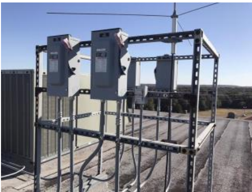
Corroded rooftop pipes
