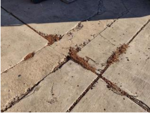
Cracked sidewalk
