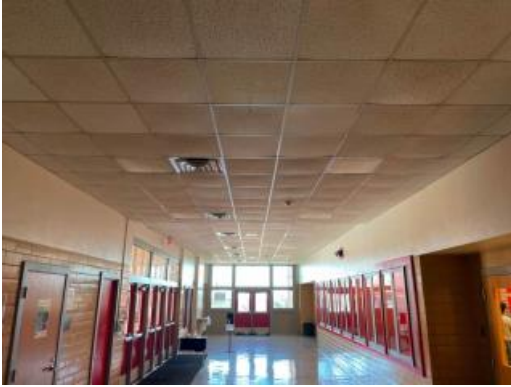
Old Acoustical Ceiling Tile
