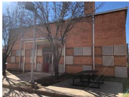
Exterior Brick walls
