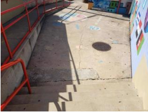
Cracked sidewalk
